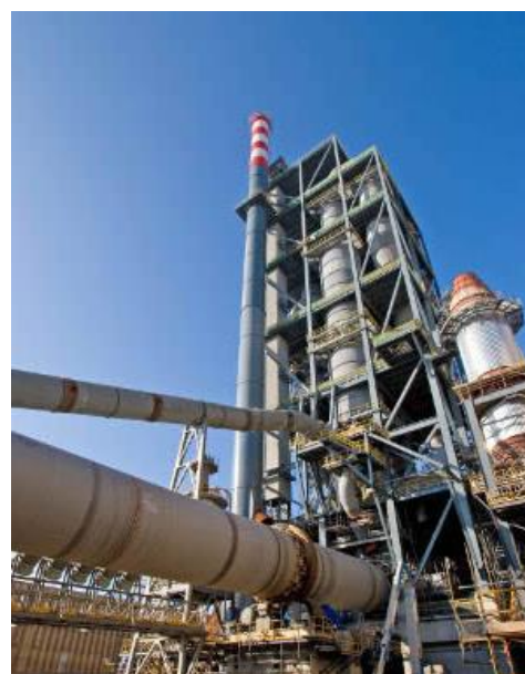
Plate 1.2 Photo of Preheater tower and Kiln 3 at Platin
